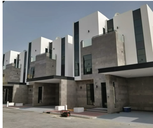
Project: G+1 Commercial Villas (8 Nos.) Shakhbout City Client: Crown Prince Court Emirates of Abu Dhabi. Main Contractor: Skyline General Contracting Est. Consultant: e11 Engineering Consultants
