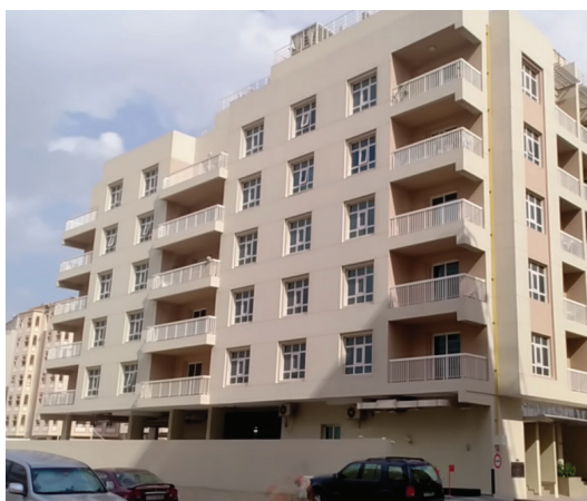
Project: G+6 Residential Building, Al Warqa Client: Hassan Mohammad Jassim Al Jassami Main Contractor: Al Hudaiba Consultant: Next Engineering Consultancy
