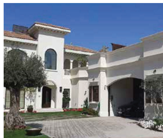
Project: B+G+1+R Private Villa, Jumeirah Golf Estate Client: Mr.Jaber Abdul Wahab (CEO-Bridgeway GOC) Main Contractor: Al Faisaliyah Contracting llc Consultant: Emarati Engineering Consultancy
