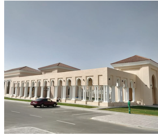
Project: Majlis at Camel Race Federation in Al Wathba, Client: H.H Sheikh Mansoor Bin Zayed Al Nahyan Eng Office Main Contractor: Civen Construction Co. Ilc - CIVENCO Consultant: e11 Engineering Consultants
