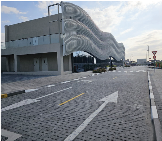
Project: TSE Pump Stn & Main Sewage Pump Stn Client: Govt of Sharjah Dept of Public Works Main Contractor: Sea Rock Technical Cont llc Consultant: Jacobs
