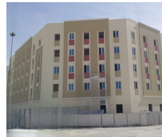
Project: G+4+R Labour Accommodation, Jabel Ali Client: Tariq Mohamed Abdulrahman Alashram Al Flassi Main Contractor: China Rail 18th Bureau Group Ilc Consultant: Future Art
